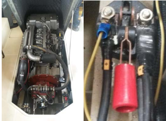
Figure 15: The main switch power distribution
